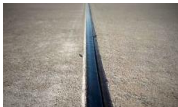
Deformation joint in concrete
