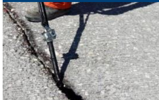
Crack sealing in asphalt
