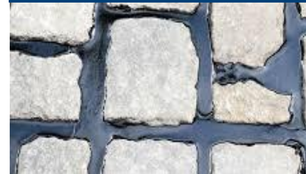
Sealing of paving stones
