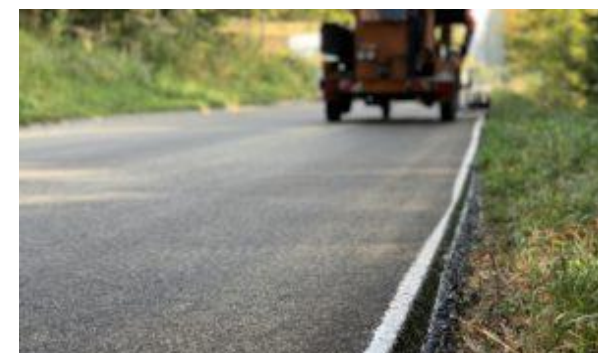
Roadside edge waterproofing
