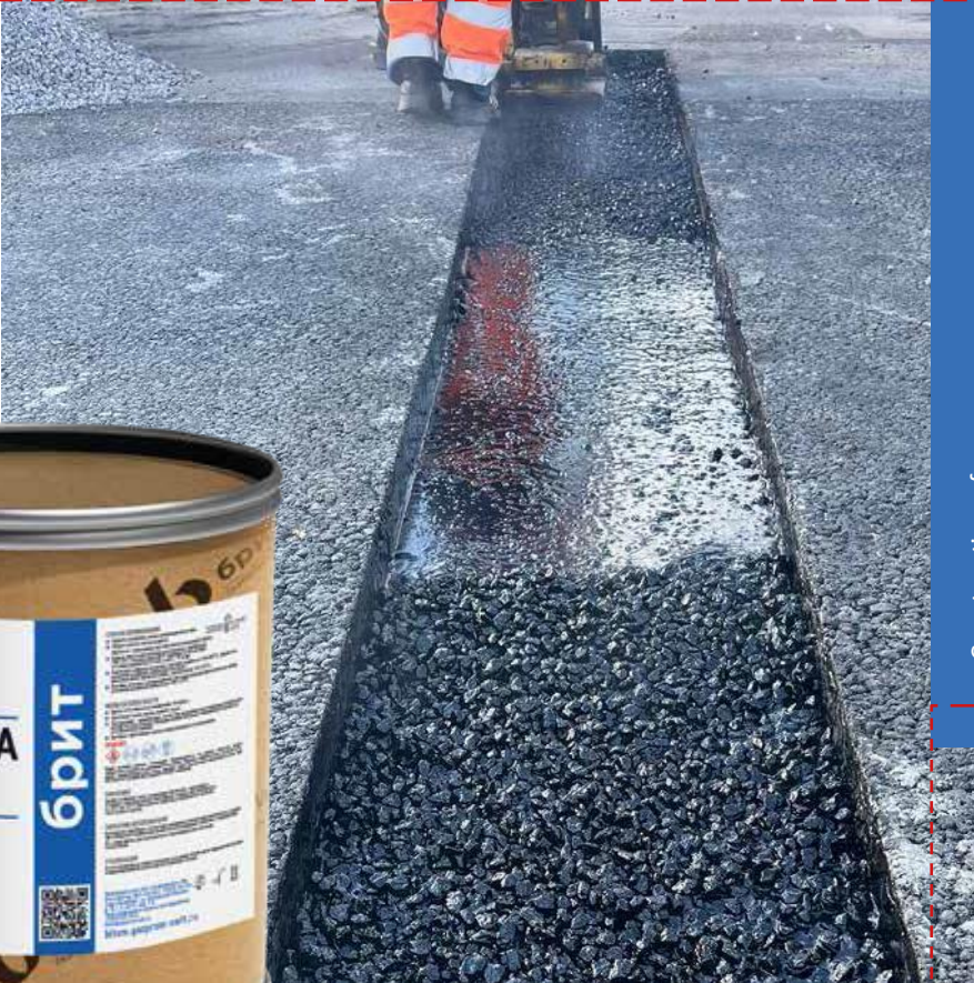
Construction of expansion joints
